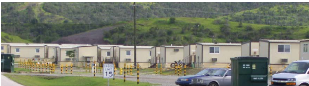
An estimated 580 troops live in containerized housing units manufactured in 2006 and 2008. All units have exceeded their economic life of five to seven years. Common problems with the units are roof leaks, plumbing failures and mold growth. (Courtesy Photo)
